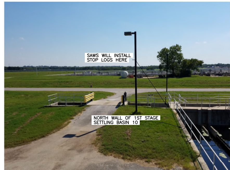
DEWATERING DISCHARGE LOCATION
